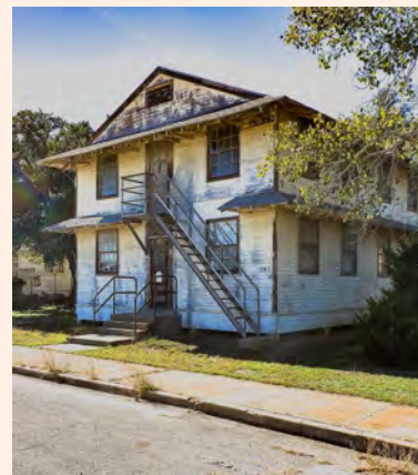
WWII Army wooden two story barracks then and what is left. There were thousands of these built, which could burn down in under four minutes and usually-house 52 soldiers at a time.
