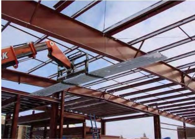
**Top photo** - depicts a section of the corrugated steel roof being hoisted into position.
